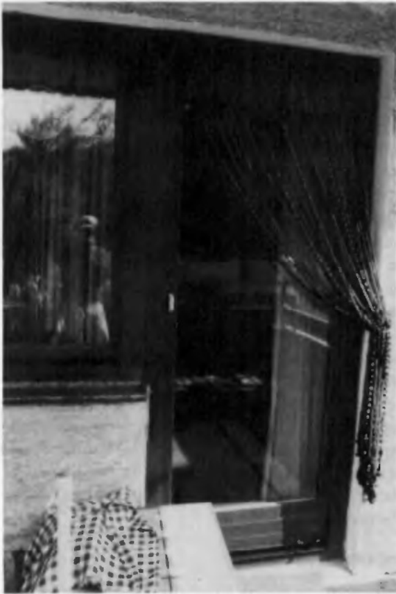
FIG. 3. (a) The original window and glass door at house 1; (b) the retrofit window and glass door at house 2.
